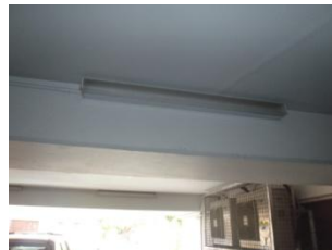
Ceiling and wall linings
