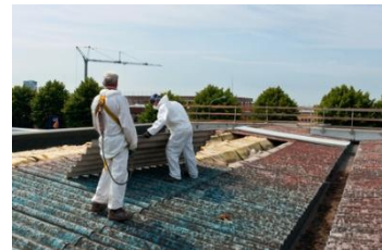
Corrugated cement roof sheeting
