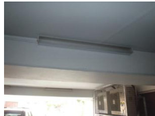
Ceiling and wall linings
