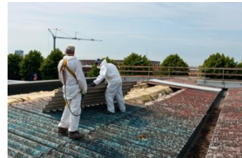
Corrugated cement roof sheeting
